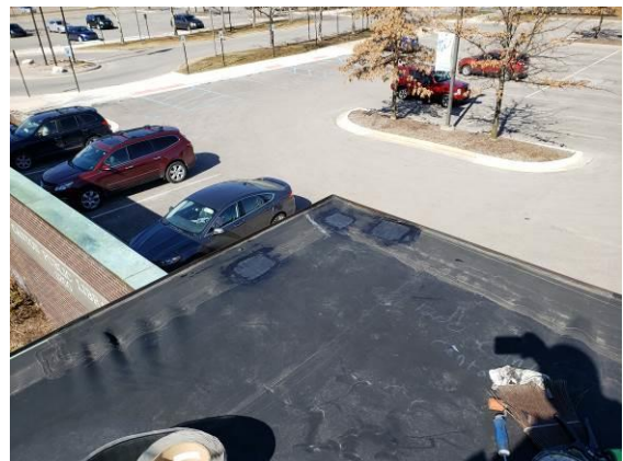
4. Intertek installed repair patches over these holes.
