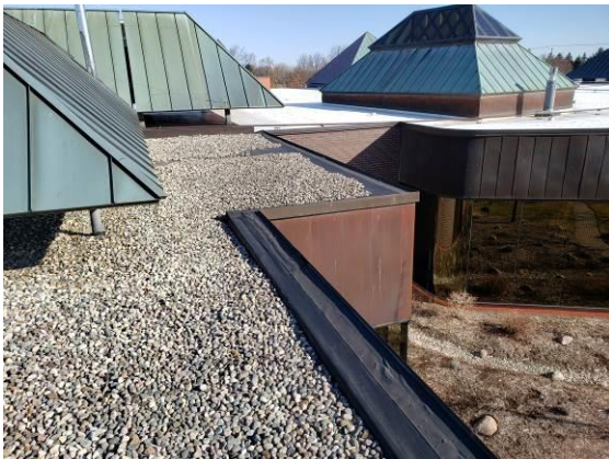
9. View of the typical raised perimeter metal edge.
