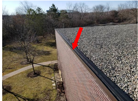
22. View of a typical roof edge.
