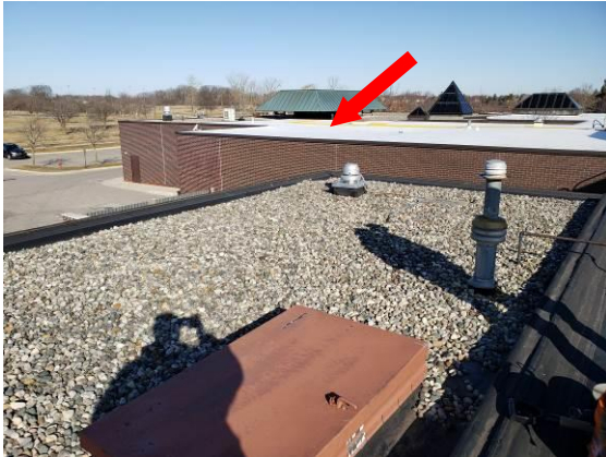
7. View of the smaller south building addition, looking northwest.
