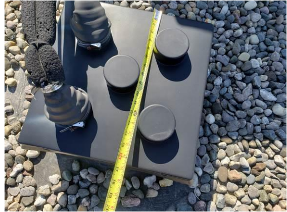
20. Typical Portals Plus cap, which may be able to be salvaged and re-used during roof renovation.
