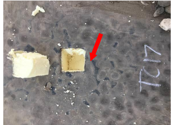
22. Photo of Test Cut #17. Insulation found dry to touch.
