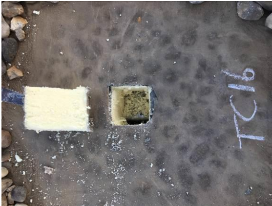
21. Photo of Test Cut #16. Insulation found dry to touch.
