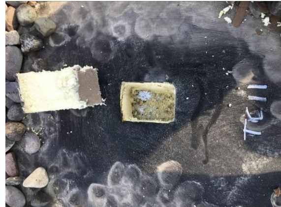
16. Photo of Test Cut #11. Insulation found dry to touch.
