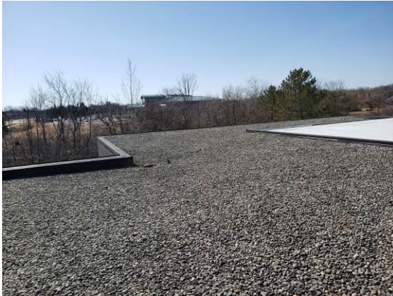
1. General view of East Area roof, looking south. Aggregate surfaced EPDM.
