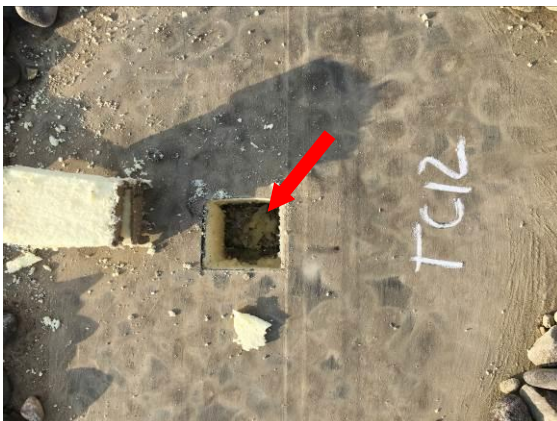
17. Photo of Test Cut #12. Insulation found dry to touch.
