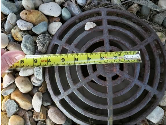
19. Typical existing 4" roof drain on the larger roof sections.
