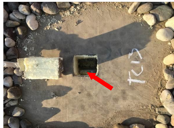
18. Photo of Test Cut #13. Insulation found dry to touch.
