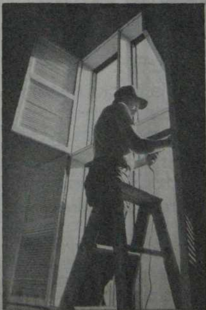
Donald Miller hangs shutters on the library building.
