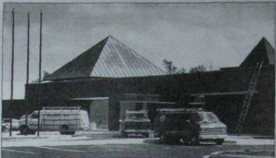
Work crews are out in full force at Canton's new library.
