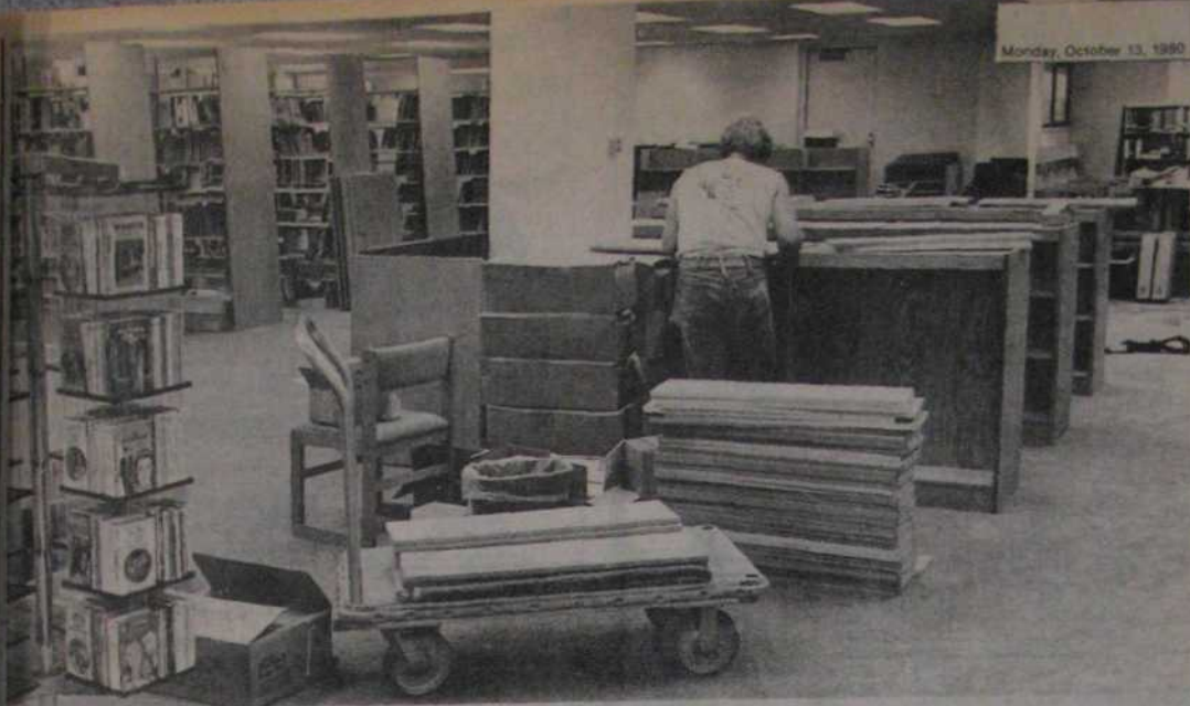
A construction worker sets up tables and shelves in the new Canton Public Library in preparation for the Oct. 20 opening. (Staff photo by Gary Caskey.)
